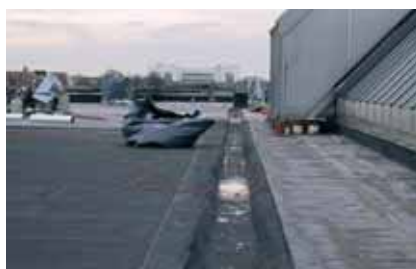
Sealing simple gutters using RESITRIX SK or classic
