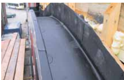
Sealing a convex curved gutter using RESITRIX SK
