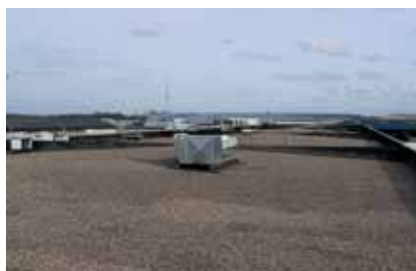
RESITRIX MB laid loose with ballast
