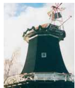
WATERPROOFING TO WINDMILL, NETHERLANDS
