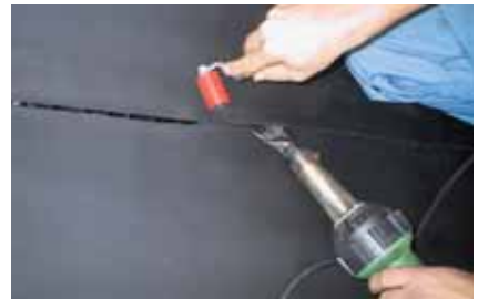
Heat welding with a handgun e.g. for corners and detail work
