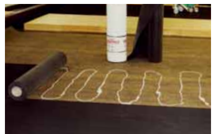
RESITRIX classic bonded with strips of PU-LMF-98 adhesive
