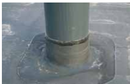
Sealing around pipe penetrations using separate pieces of RESITRIX SK or classic
