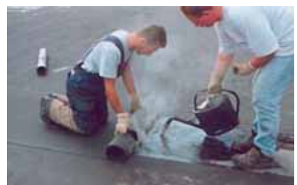
RESITRIX classic fully bonded in hot bitumen
