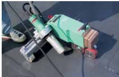
Machine welding laps in self-adhesive RESITRIX SK using a 40 mm wide nozzle
