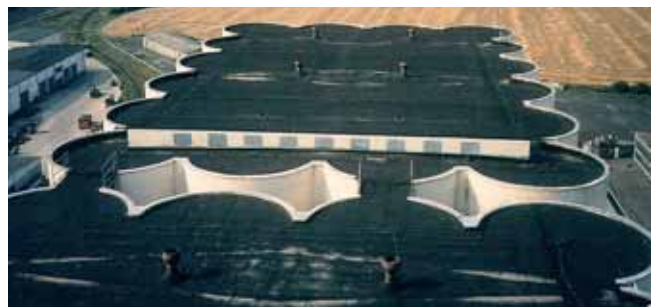
STORAGE SILOS, KARSTÄDT
