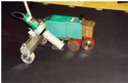
Heat welding mechanically fixed RESITRIX MB using a Leister Varimat with 85 mm wide nozzle
