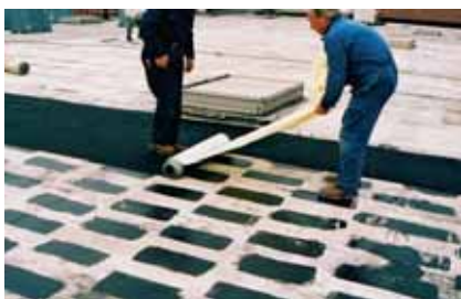
Partially bonding RESITRIX SK after partial application of FG 35 primer
