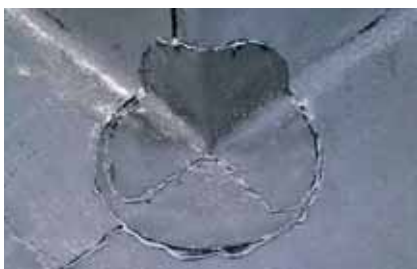
Site-formed external corner using separate pieces of RESITRIX SK, MB or classic
